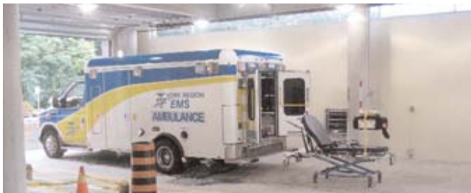
The Nick and Rosanne Cortellucci Family Emergency Department also includes a heated, ambulance bay capable of handling up to four vehicles.
